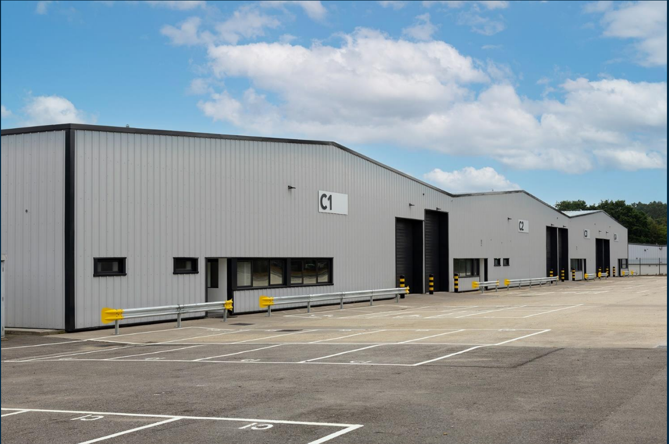
Units C1-C4, Woolborough Lane IE, Crawley
